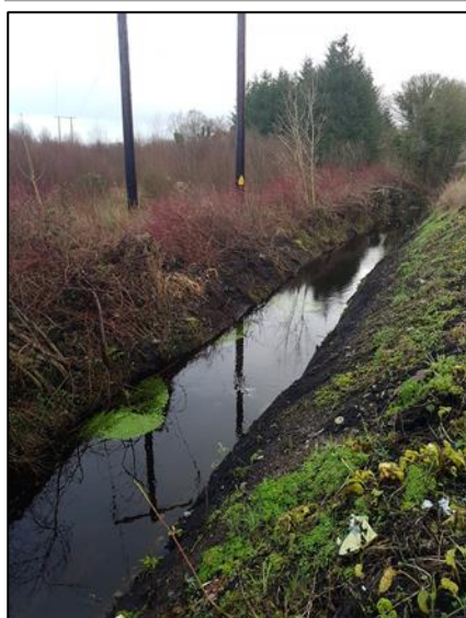
Water crossing 3; FW4 Drainage ditch
