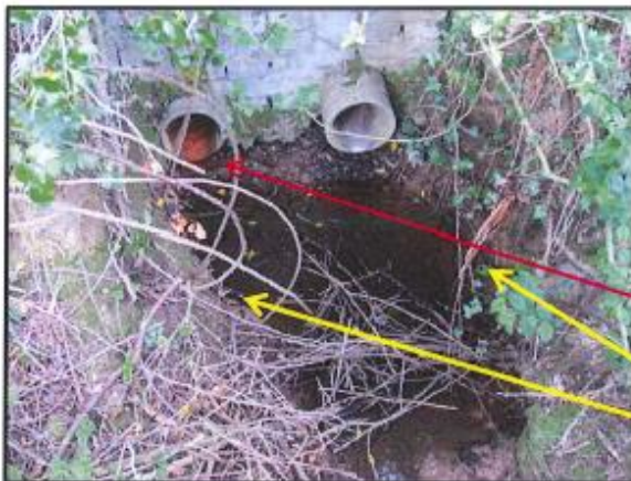
Photo 5. W34a. This is a small watercourse that was identified as we were leaving this area. It appears that there is a small amount of flow on the left-hand channel. The flow is seasonal. There is evidence of erosion under the pipes. IFI recommend that after the cable is laid that the bed is backfilled with crushed rock to a point level with the lowest pipe. It may also be necessary to put small amount of light cobble as rock armour against the clay banks on either side. If this bridge is being replaced a 900mm diam. pipe would be the minimum requirement.
